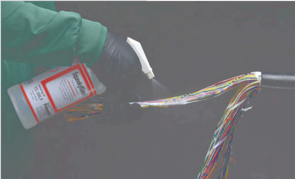
TC-35LR cleaning 200-pair copper cable
